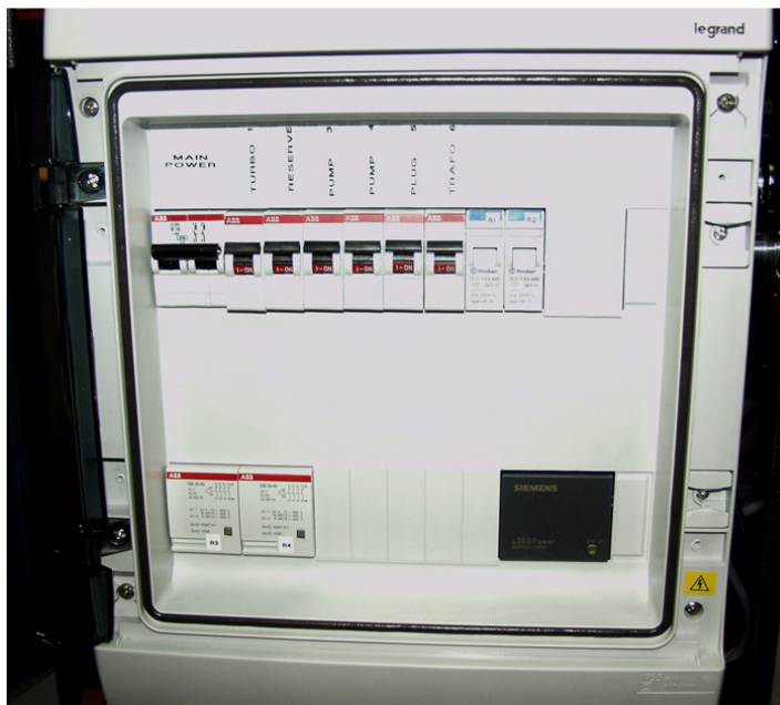
Fig 13 Main relay box
